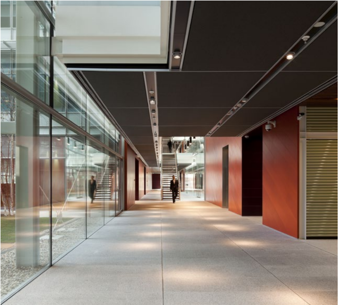
covering: natural stone panel core: calcium sulphate dimensions: special size
