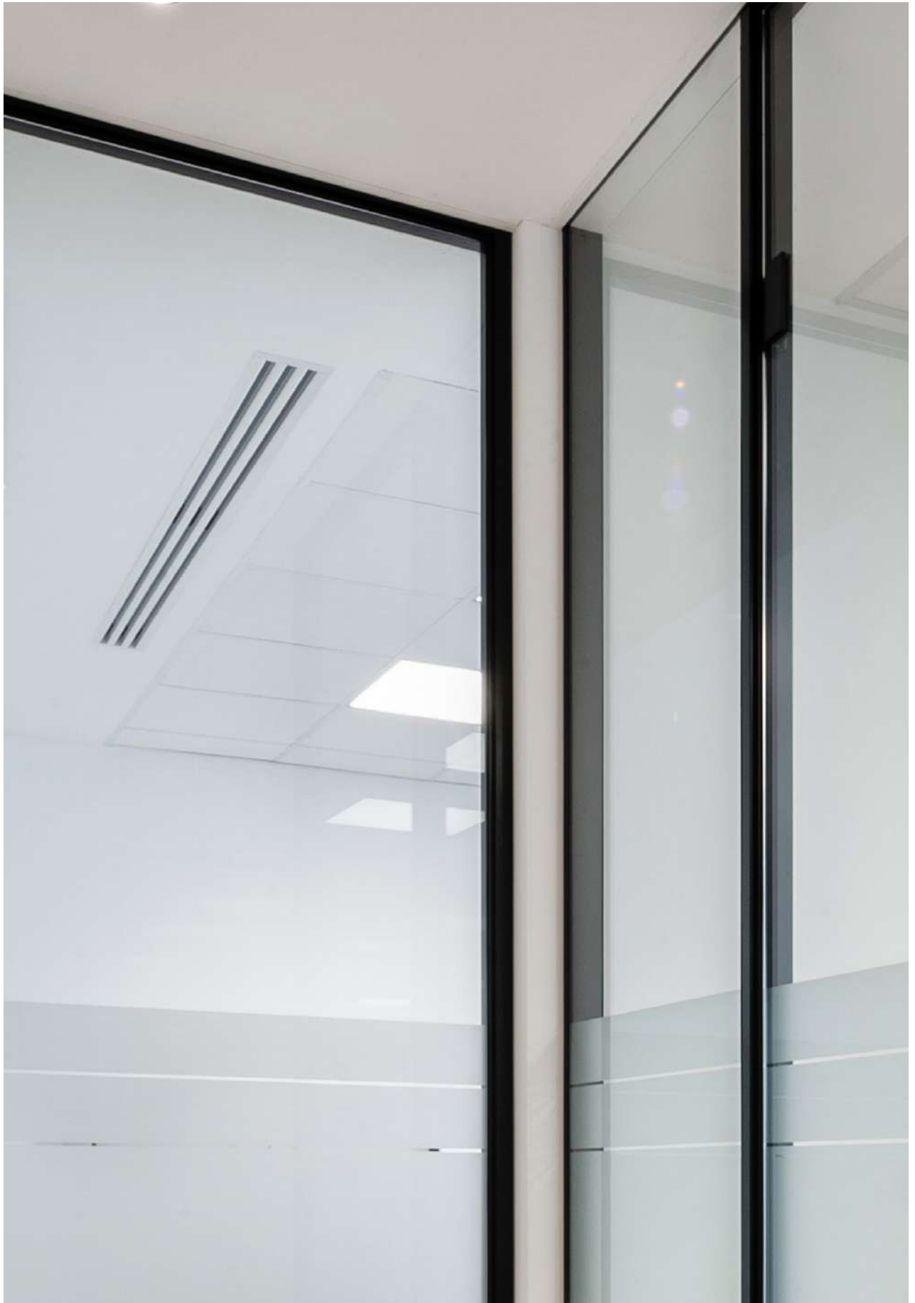
HEADQUARTER IN PADOVA /RADIANT CEILING
