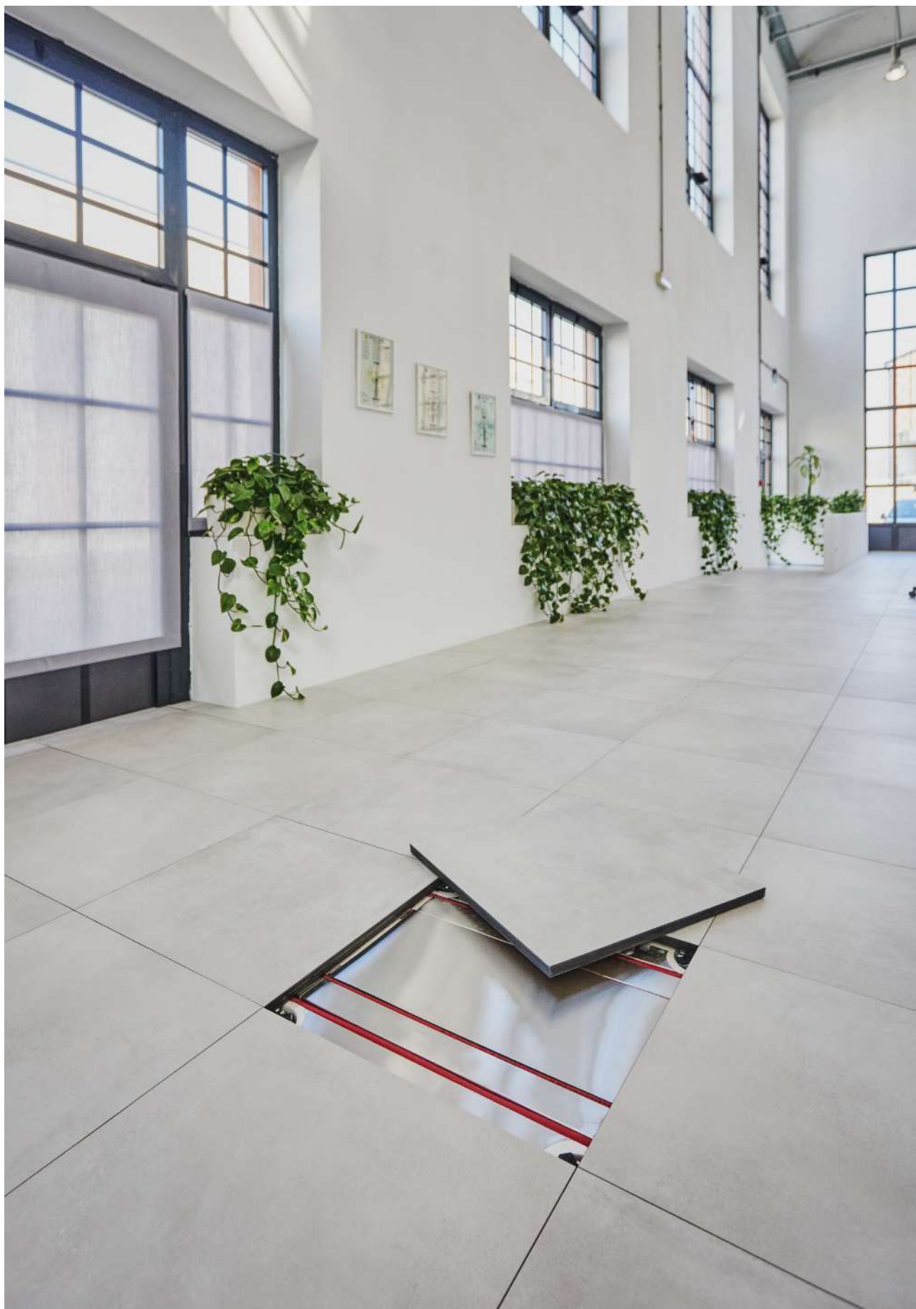
HEADQUARTER IN ROVIGO /INSPECTIONABLE RADIANT FLOOR
