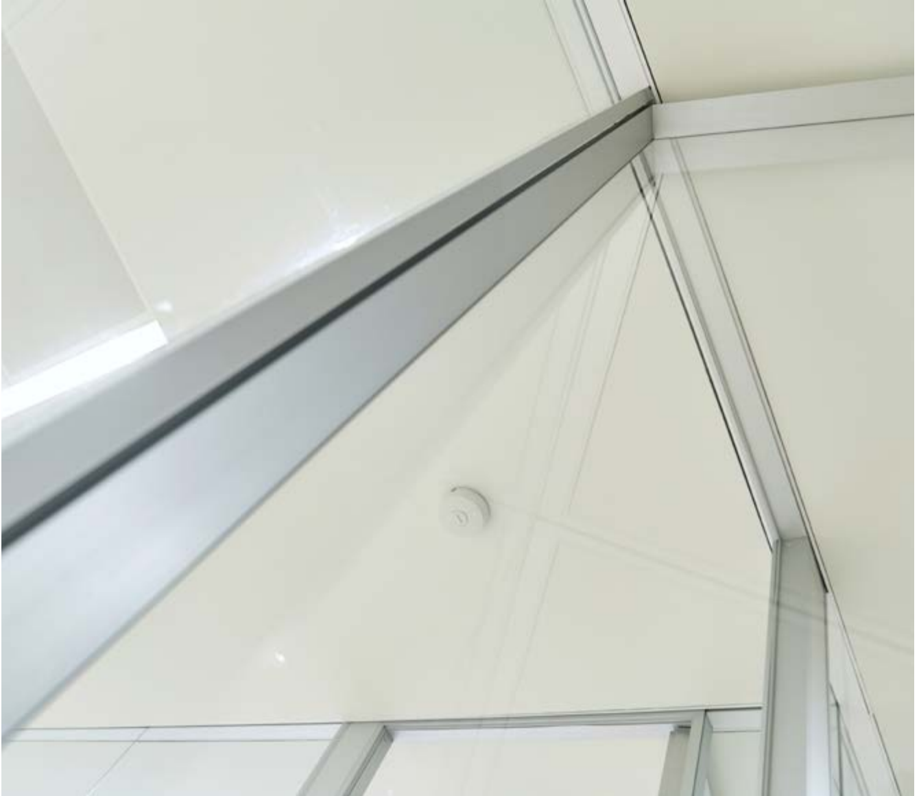
detail of glass partition integrated into the ceiling
