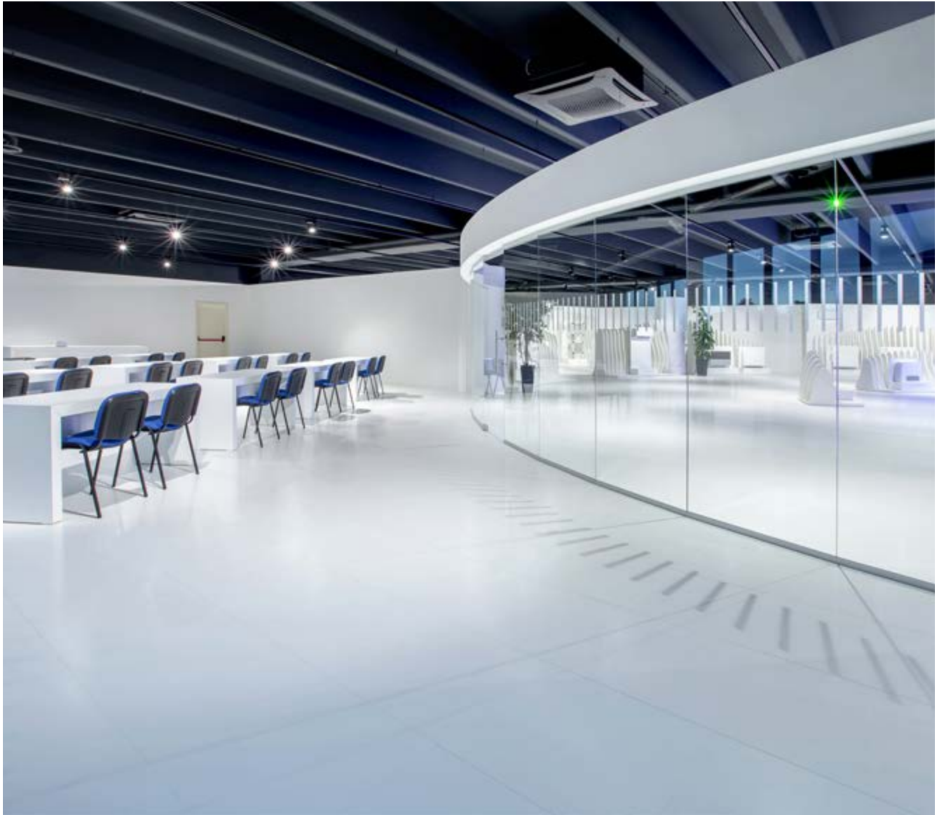
covering: white (RAL 9003) resin panel core: calcium sulphate dimensions: 600x600 mm
