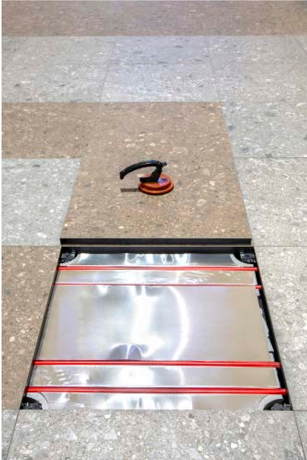
DIFFUSE radiant system covering: ceramic dimensions: 600x600 mm
