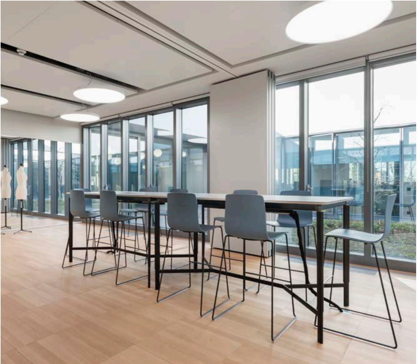
covering: oak panel core: calcium sulphate dimensions: 600x600 mm
