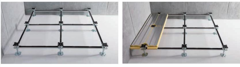
3/ Complete the laying of "active" panels on all the pedestal rows.
